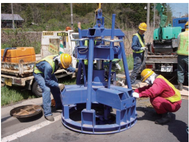
During construction (removal of a manhole)
