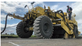
Construction with a road stabilizer
