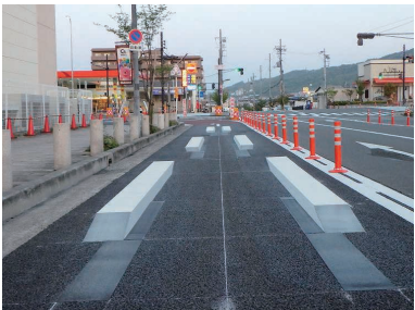
Road markings that appear to be three-dimensional
